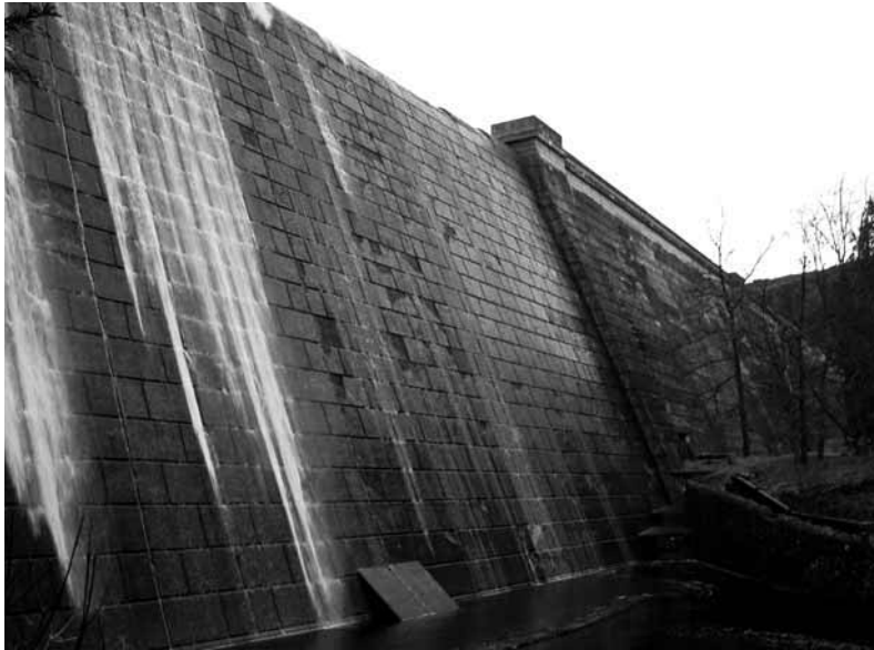
Haweswater, Lake District. This 470-metre-long dam is unusual, being a concrete buttress dam, but the 44 buttresses are widened at their end so that the dam's air face, while appearing uniform, is in fact hollow, comprising a series of linked pyramid chambers, thus saving concrete.
