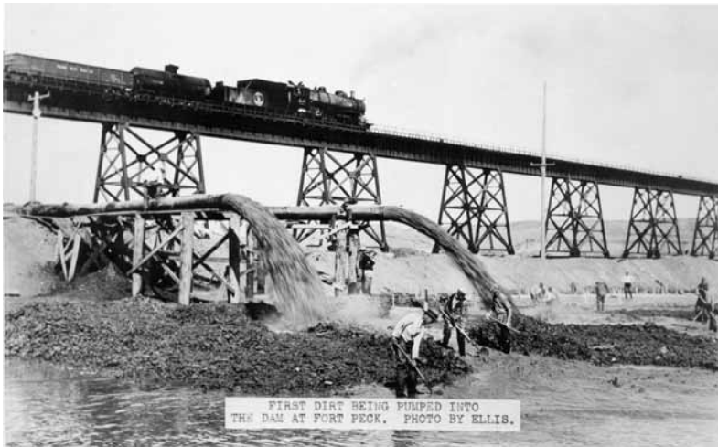
'First dirt being pumped': Fort Peck Dam on the Missouri River, Montana. The largest hydraulically filled dam in the USA, completed in 1940.
