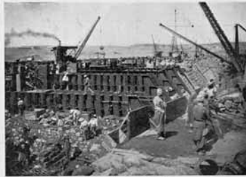
Composite Metal and Masonry Construction, Assouan.
