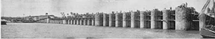
Nile Reservoir Works, Assiut—Upstream Side of Piers, Looking West.
