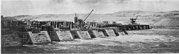
Assouan Dam—Water Rushing Through Central Spikes.
