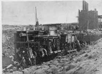
Centrifugal Pumps at the Foundation Excavations.
